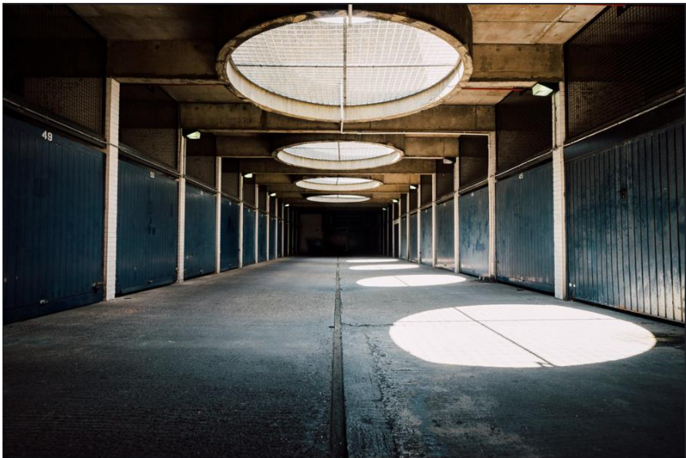
Parking and garaging below. Note the striking presence of sunlight through the circular lights.
