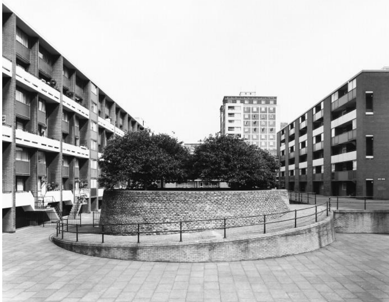
Looking east between Basterfield House (L) and Bayer House (R)
