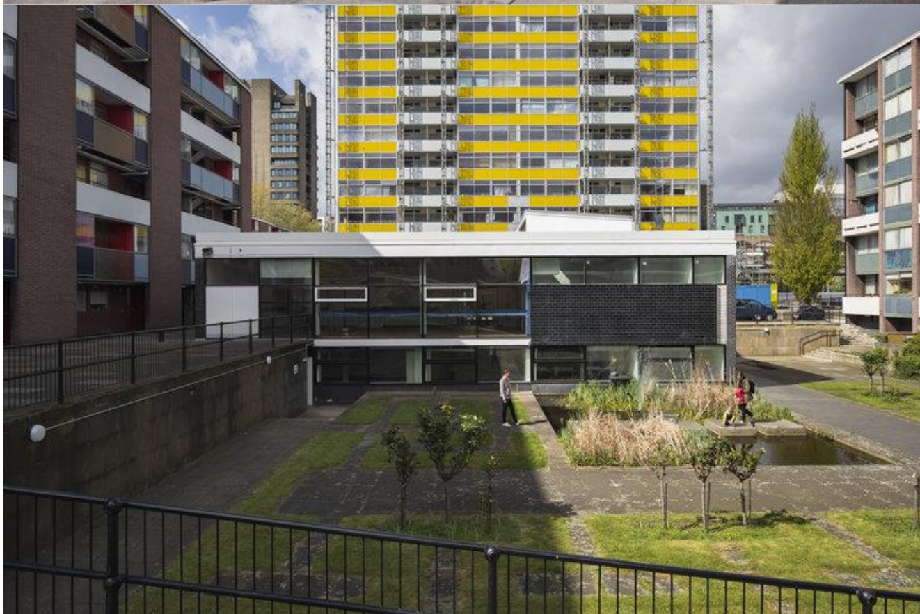
Two views, historic and modern, looking west at the Community Centre with Great Arthur House in the background
